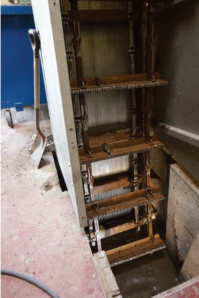
Channel modifications were required.
